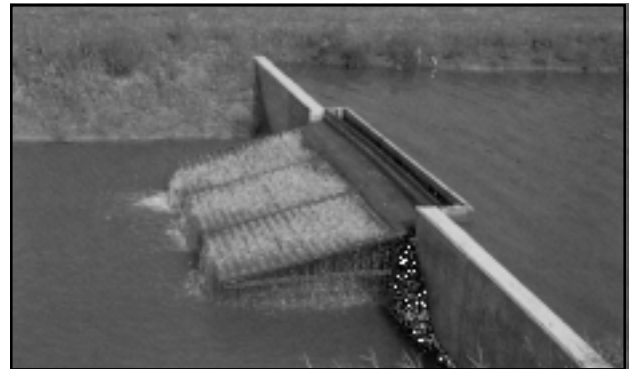
Figure 2. Gravity aerator in a recirculating raceway system.
