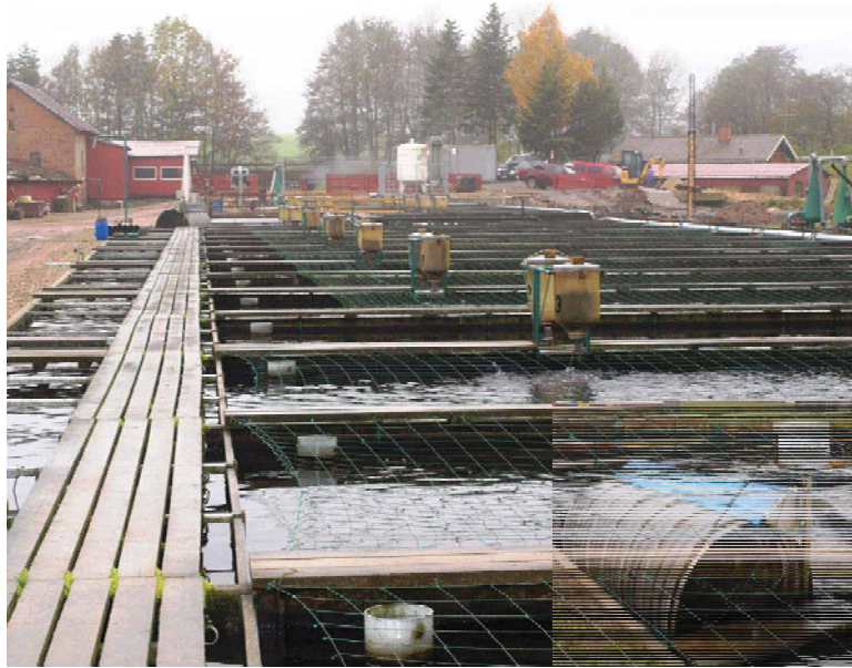
Figure 12. Bregnholm Mølle Model Trout Farm (type 1) with a micro sieve inserted in the right corner. Photo: Lisbeth J. Plesner.
