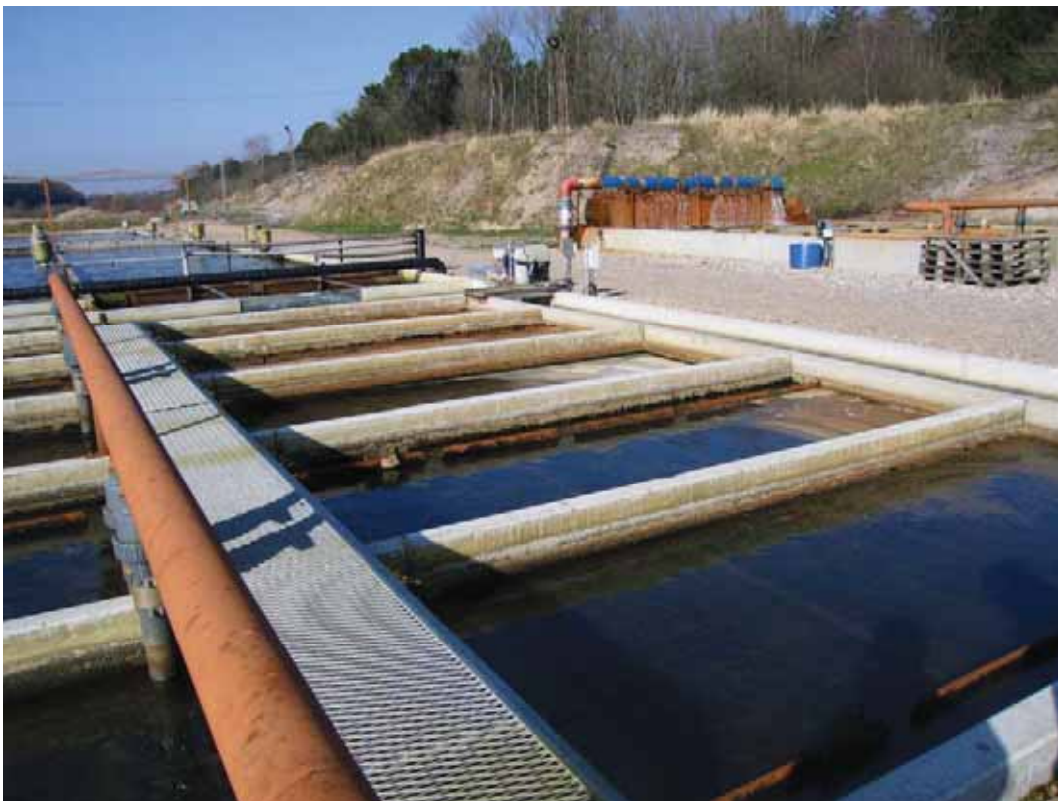
Figure 20. Biofilter divided into sections with bio blocks at Ejstrupholm Model trout farm (type 3). To the right of the biofilters is an ochre device for aeration of the abstracted ground water and precipitation of the ochre before the water enters the production units. Photo: Alfred Jokumsen.
