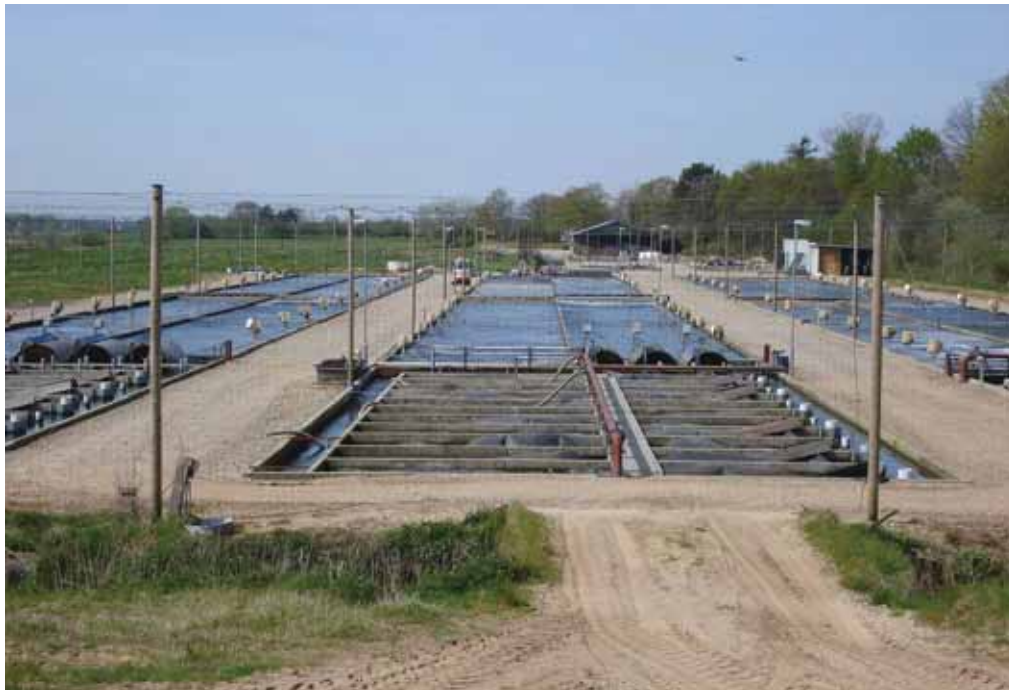
Figure 14. Kongeåens Model Trout Farm (type 3). The production units include three sections, each consisting of two concrete raceways with micro sieves (mesh size 74 µm) in front of the biofilter sections (foreground). In the background to the left, the plant lagoons consisting of the former earthen ponds and the inlet and outlet channels are visible (Svendsen et al., 2008). Photo: Lars M. Svendsen.
