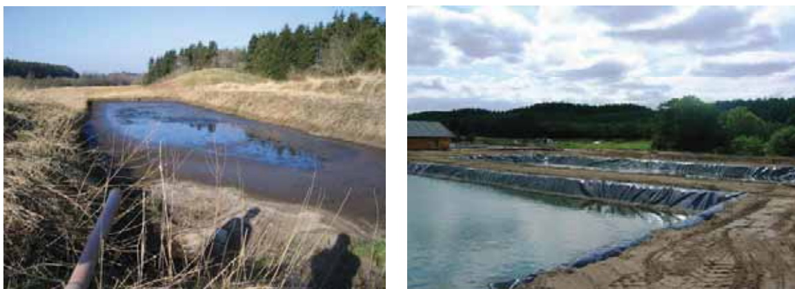
Figure 19. From the sludge cones, the sludge is transferred to sludge basins/tanks for settling of particulate matter. Left from Ejstrupholm Model Trout Farm (Photo Alfred Jokumsen) and right from Løjstrup Model Trout Farm. Photo: Lisbeth J. Plesner.
