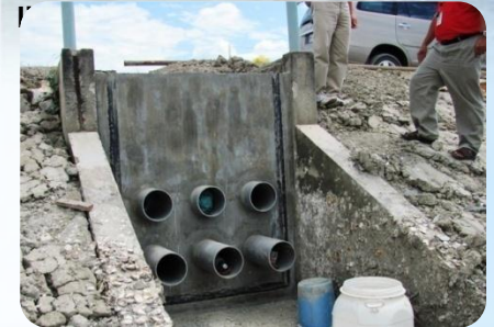
Pond outlet gate
