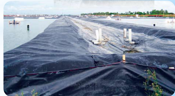
HDPE Lined secondary supply canal
