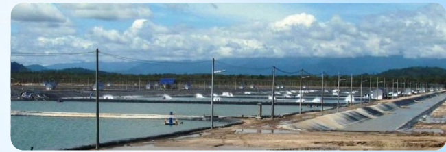
RAS iSHARP modules, Malaysia
