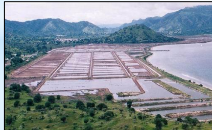
Flow through + WWST, Sumbawa, Indonesia
