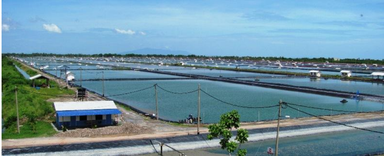
HDPE lined ponds with center drain, secured outlet gates & Main supply canal
