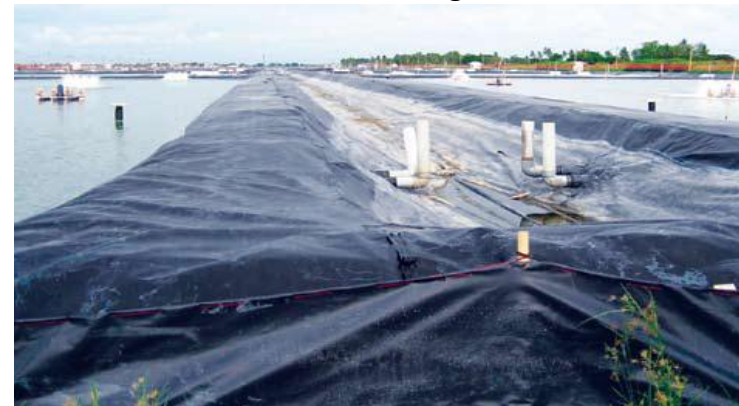
HDPE Lined secondary supply canal
