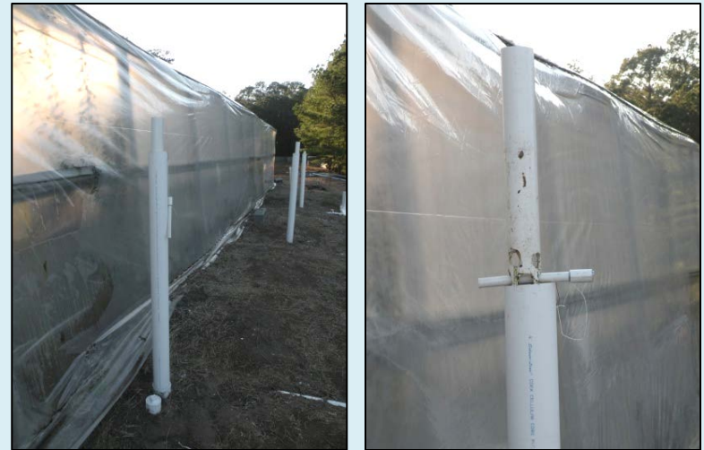
External standpipes removed daily to flush solids to shrimp tanks.
